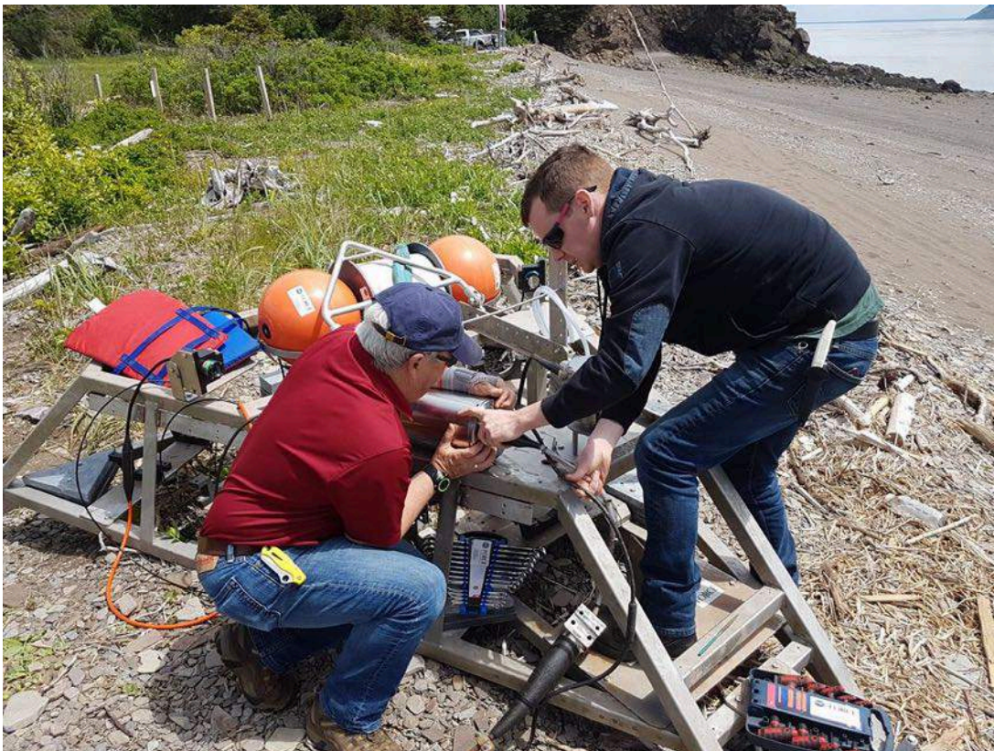
Figure 12: FORCE personnel work on the FAST-2 sensor platform in mid-June, connecting a multibeam imaging sonar camera to a multiplexer, which collects and transmits data to shore via optical fibres.
