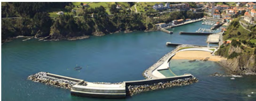
Figure 5.4. The Mutriku Wave Power Plant opened in July 2011 and provides harbor protection while generating electricity by harnessing air compressed by the action of waves, showing a positive benefit of MRE devices. The plan has 16 turbines with a total capacity of 296 kW (Ente Vasco de la Energía, http://www.eve.eus/Proyectos-energeticos/Proyectos/Energia-Marina.aspx?lang=en-GB ).
