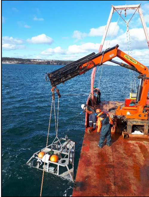
Figure 2: Deployment of the FAST platform in Grand Passage for an assessment of PAM instrument performance.
