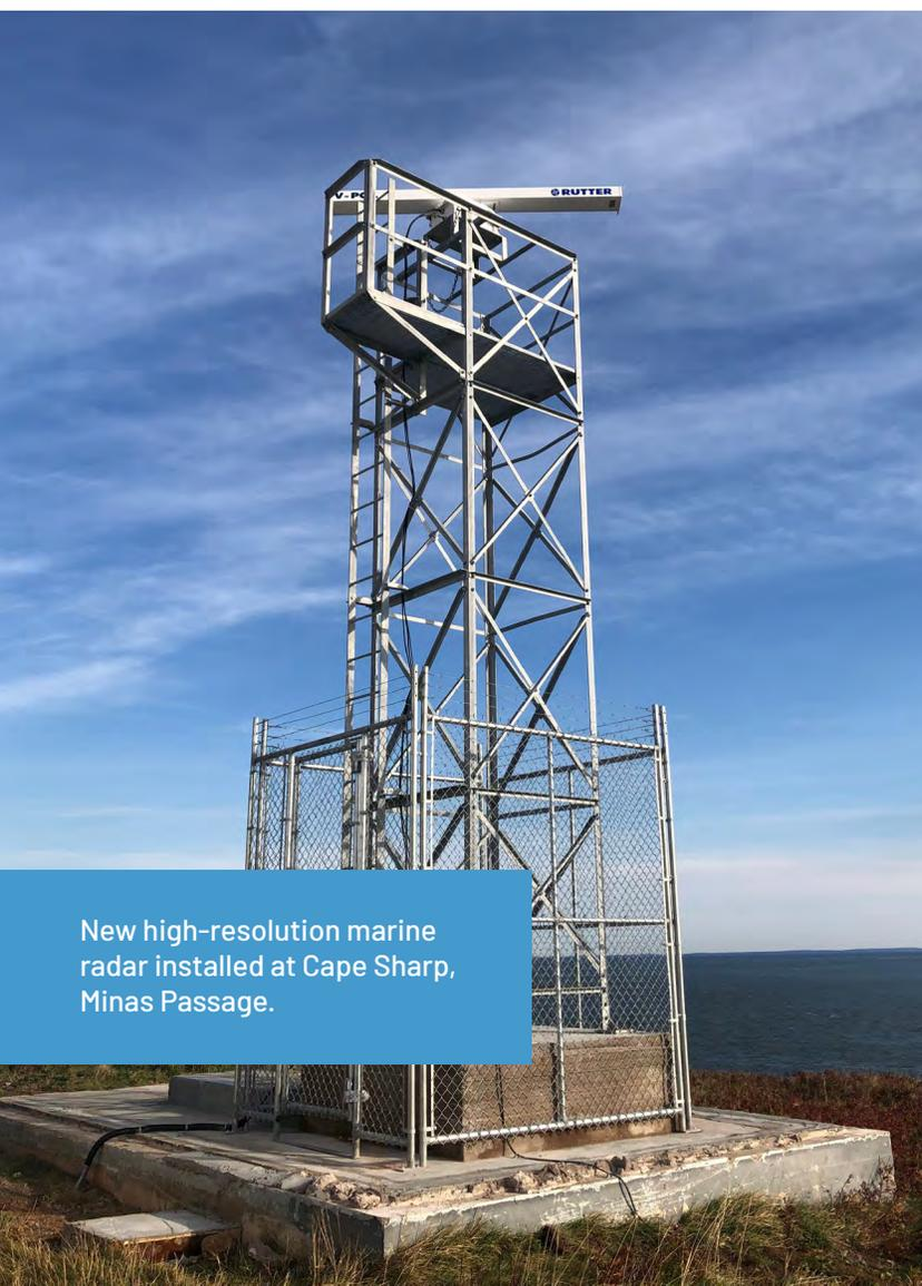
New high-resolution marine radar installed at Cape Sharp, Minas Passage.
